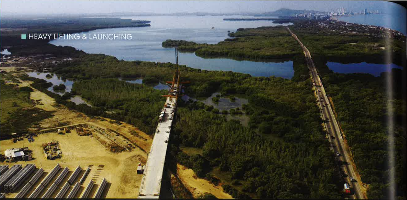
The new bridge goes through a nature reserve
