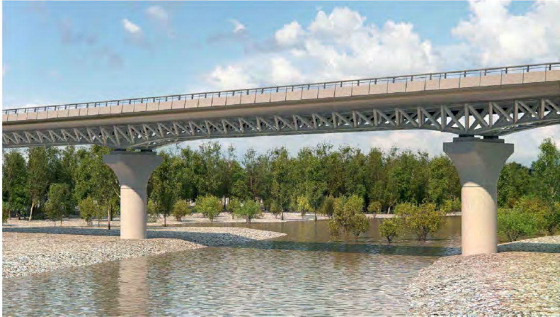
Fig. 4. New Torre Bridge rendering; the bridge has the pillars based on annular monoblock foundations
